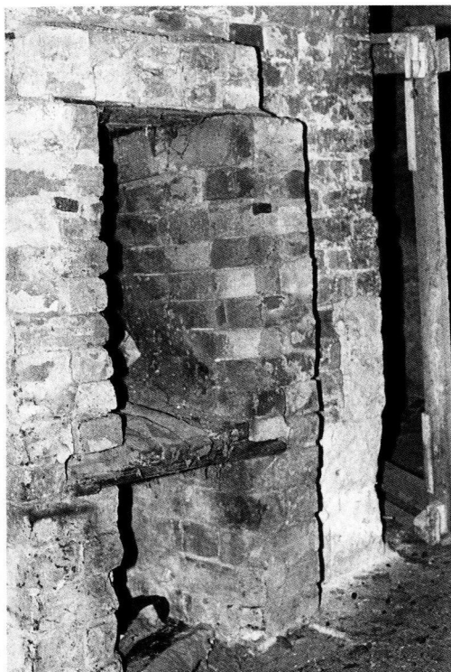
Fig. 10 (top left) Brockhampton (Glos.), The Old Brewery, the kiln furnace mouth with fire bars in a position slightly below midway. Photograph, author 1995
