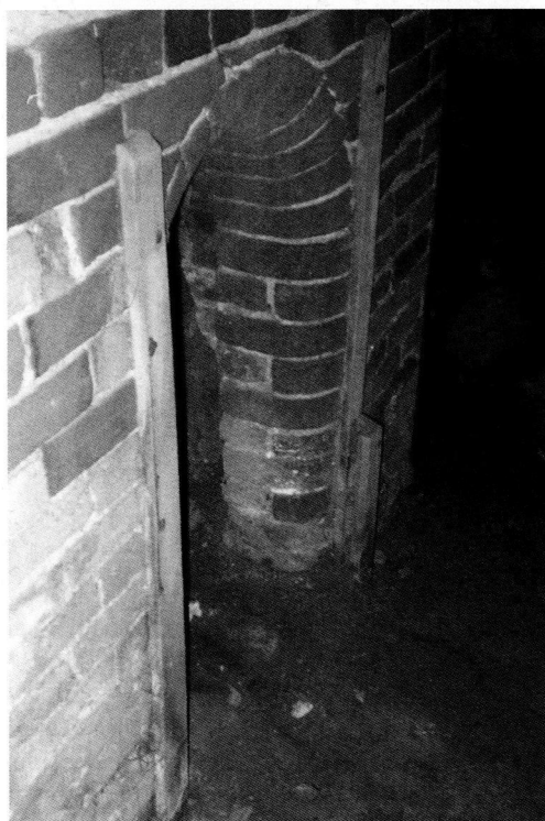
Fig. 10 (top left) Brockhampton (Glos.), The Old Brewery, the kiln furnace mouth with fire bars in a position slightly below midway. Photograph, author 1995
